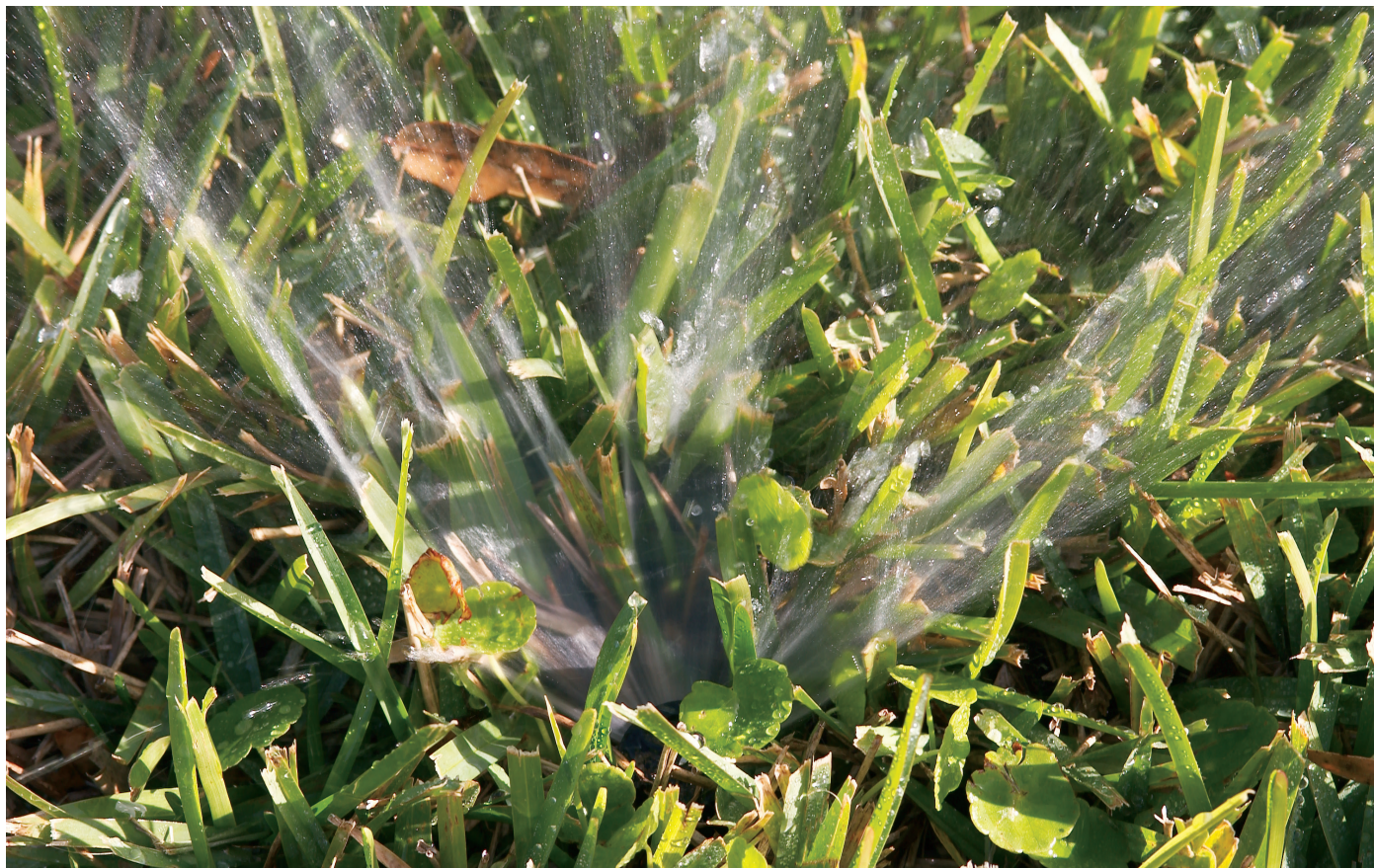
Without proper maintenance, spray heads can become too low to the ground to be effective, such as this example. Use six-inch pop-up riser extensions and periodically raise spray heads above grass beds.
