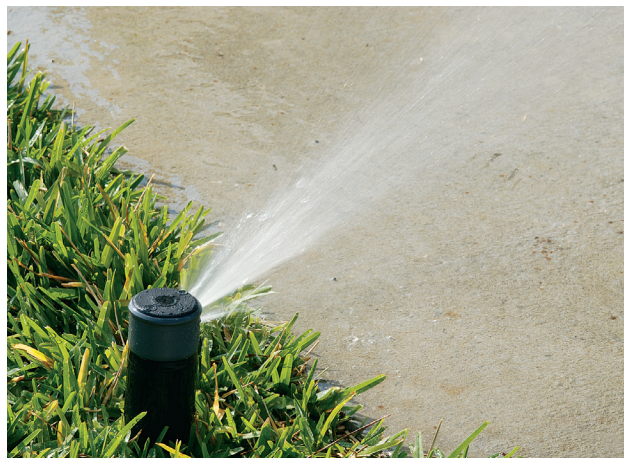
Sprinkler heads that are not adjusted can waste water by spraying onto paved areas.
