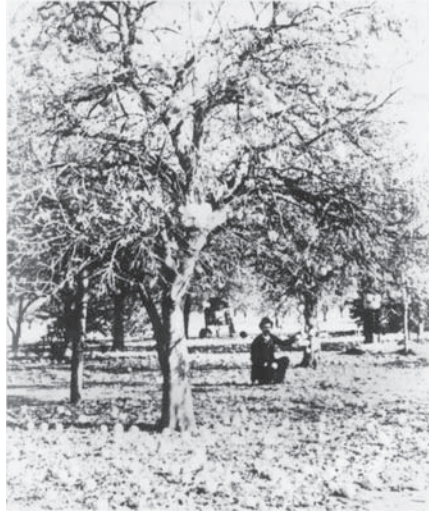
Frost damage to citrus crop
