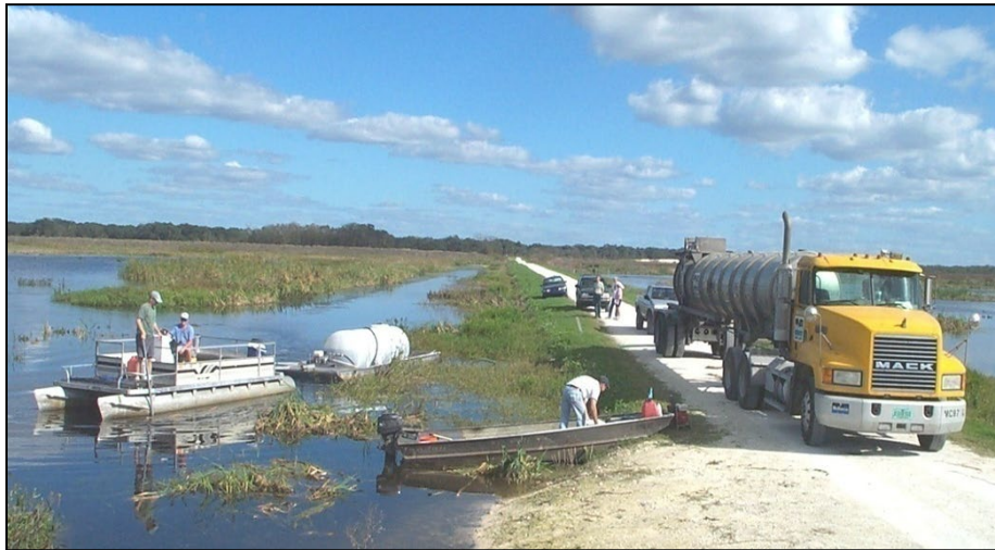
Figure 5. Alum tank being pulled on a floating barge behind a pontoon boat.
