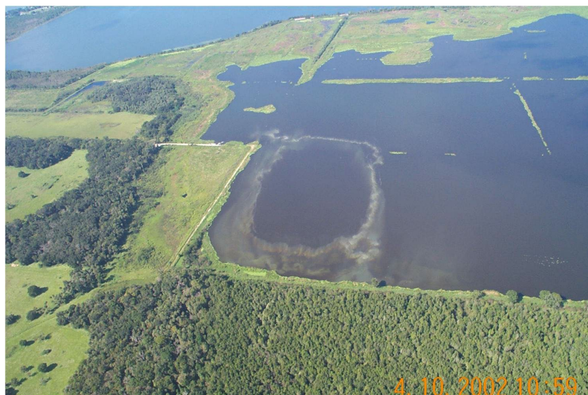
Figure 10. Aerial view of Lowrie Brown alum application. Lake Griffin visible in upper left corner.
