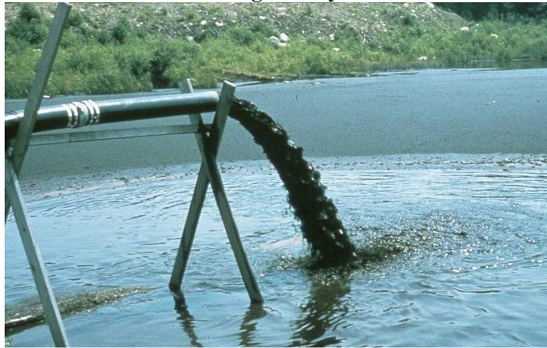
Another advantage of rapid dewatering is the enhancement of the quality of water returned to the waterbody (or watershed) following the separation of water and solids. For example, the use of flocculants and coagulants can bind metals, nutrients and other pollutants to the settled solids, resulting in improved water quality of the return water.
