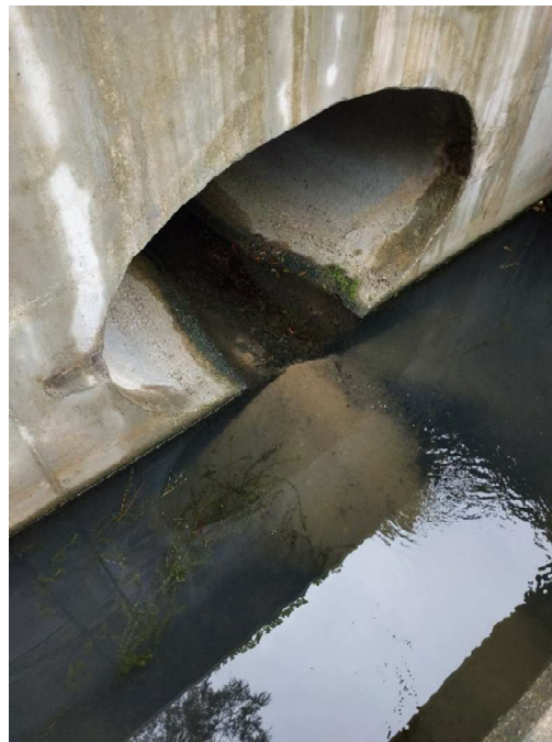
Figure 3: Sediment accumulation in sedimentation basin located at the end of the outfall pipe from the I4 runoff.
