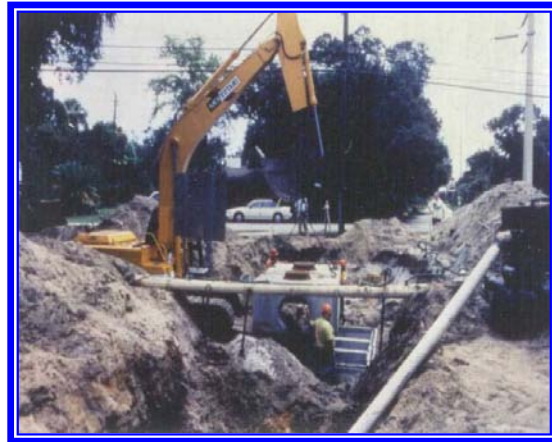
Installing a baffle box: traps soil and debris in urban runoff
