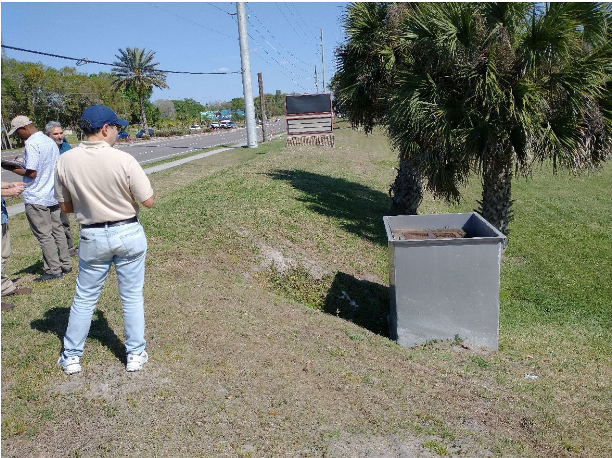
Photograph 4. A drop structure in dry detention pond from 28^{\circ} 33' 2.9'' N 81^{\circ} 36' 13.8'' W, looking east along West Colonial Drive on March 3, 2022.
