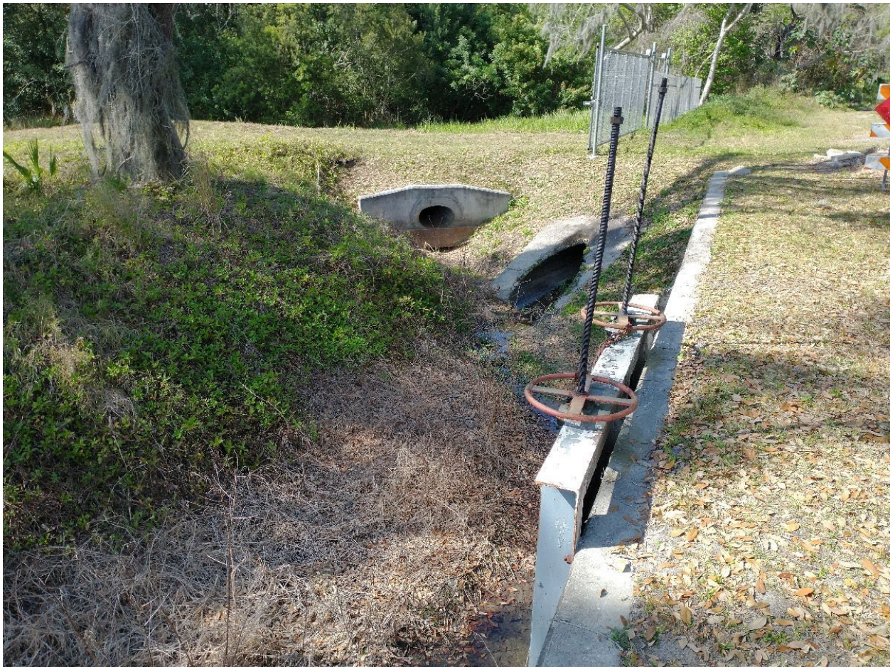
Photograph 13. Two culverts, at a water control structure (photograph 7) from 28^{\circ} 33' 5.5'' N 81^{\circ} 37' 13.5'' W, looking northwest along the southern face of the water control structure on March 3, 2022. The water control structure once regulated the flow of water from the Johns Lake watershed to a ditch that drains to Lake Apopka.
