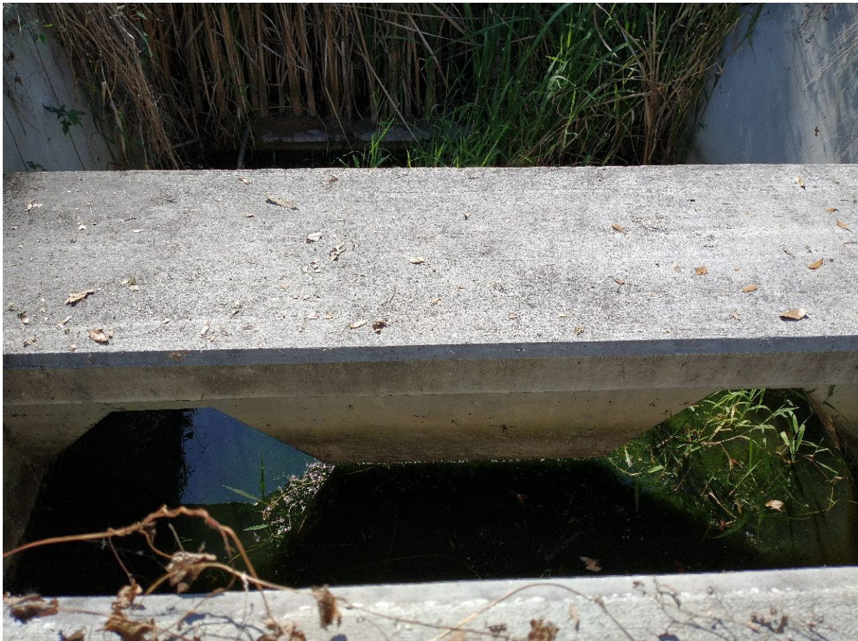
Photograph 15. A velocity damper inside a water control structure downstream of a culvert (photograph 14) from 28° 33' 29.1" N 81° 36' 59.0" W, looking down on March 3, 2022. The culvert may drain a relatively new residential development north of and outside the delineated Johns Lake overland flow simulation domain, into the domain.
