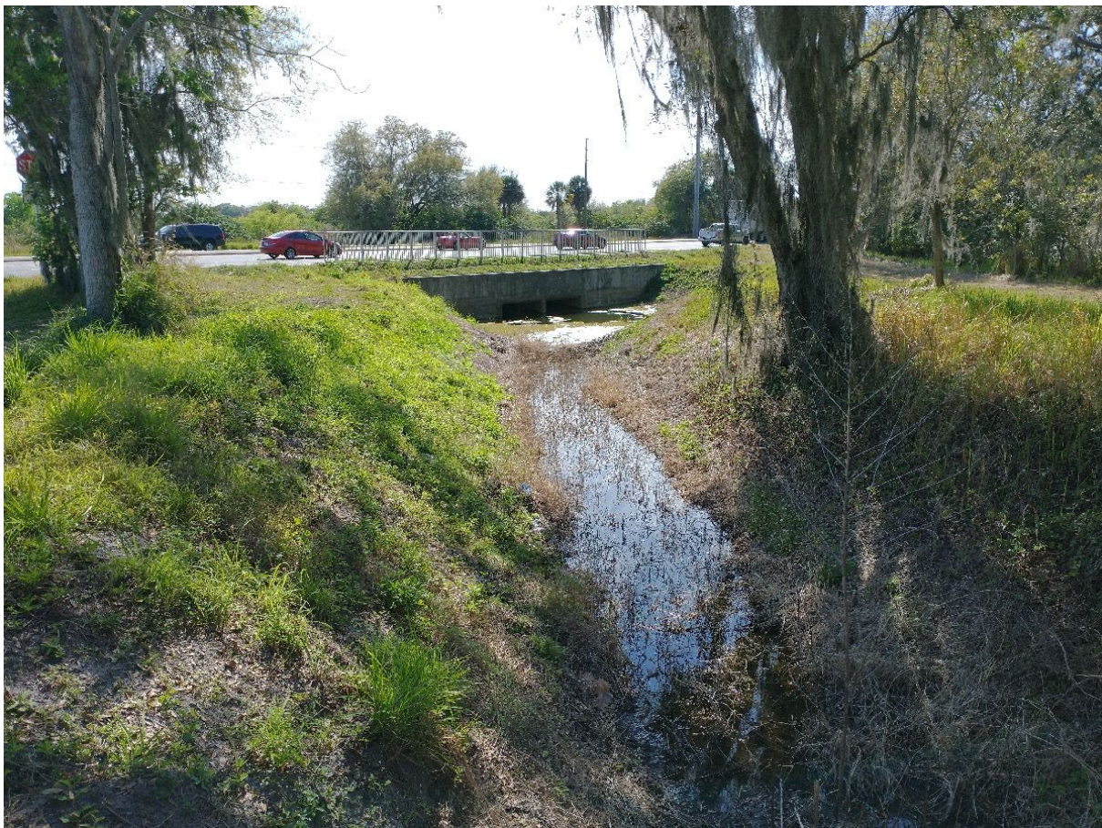
Photograph 12. A ditch and concrete apron—which functions like a weir—downstream of a twin box culvert under West Colonial Drive (photograph 10), at a water control structure (photograph 7) from 28^{\circ} 33' 5.5'' N 81^{\circ} 37' 13.5'' W, looking southwest toward West Colonial Drive and Johns Lake on March 3, 2022. The water-control structure once regulated the flow of water from the Johns Lake watershed to a ditch that drains to Lake Apopka.
