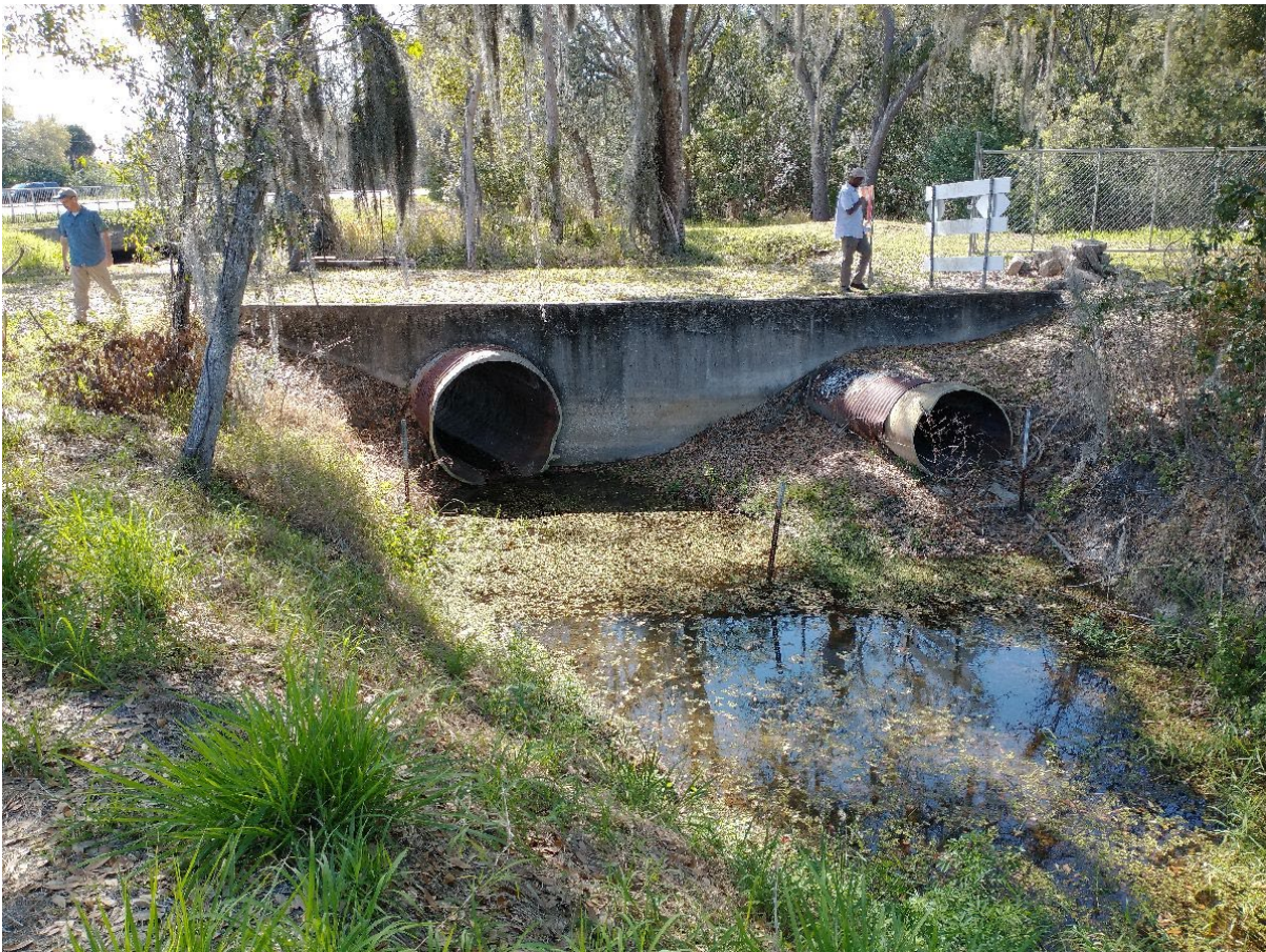
Photograph 7. The downstream side of a water control structure that once regulated the flow of water from the Johns Lake watershed to a ditch that drains to Lake Apopka, on the southeastern bank from 28° 33' 5.9" N 81° 37' 12.8" W, looking southwest toward West Colonial Drive on March 3, 2022.
