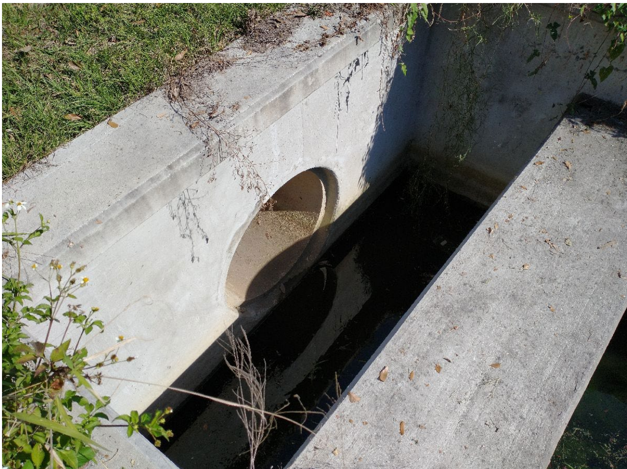
Photograph 14. The downstream side of a culvert and the top of a velocity damper inside a water-control structure, looking down and east from 28^{\circ} 33' 29.1'' N 81^{\circ} 36' 59.0'' W on March 3, 2022. The culvert may drain a relatively new residential development (photograph 17) north of and outside the delineated Johns Lake overland flow simulation domain, into the domain.
