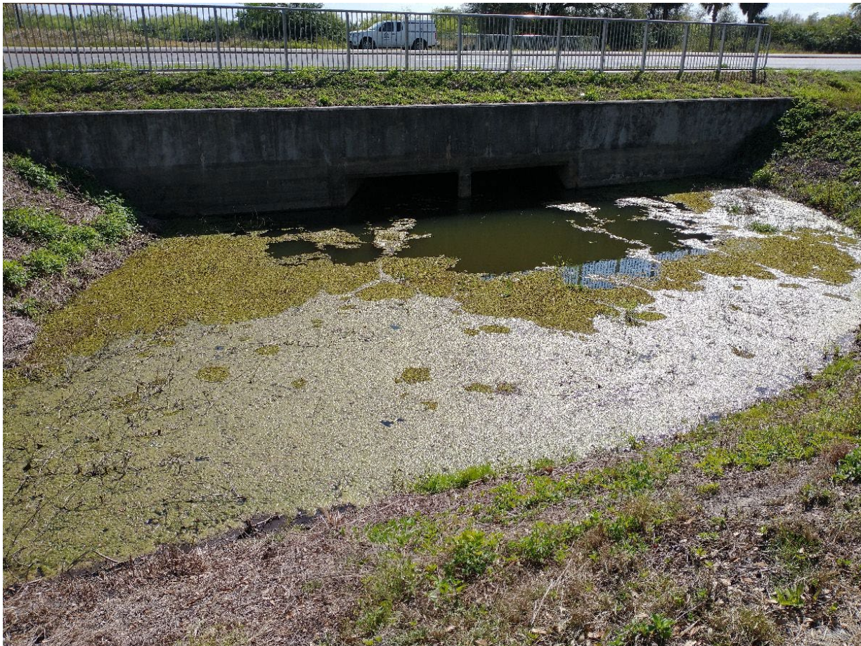
Photograph 10. The downstream side of a box culvert under West Colonial Drive from 28^{\circ} 33' 5.2'' N 81^{\circ} 37' 14.3'' W, looking southwest from the northeastern edge of a concrete erosion-control apron (photograph 11) that functions as a weir, controlling the flow of water from the Johns Lake watershed, toward a former water control structure (photograph 9), to a ditch that drains to Lake Apopka (photograph 8) on March 3, 2022.
