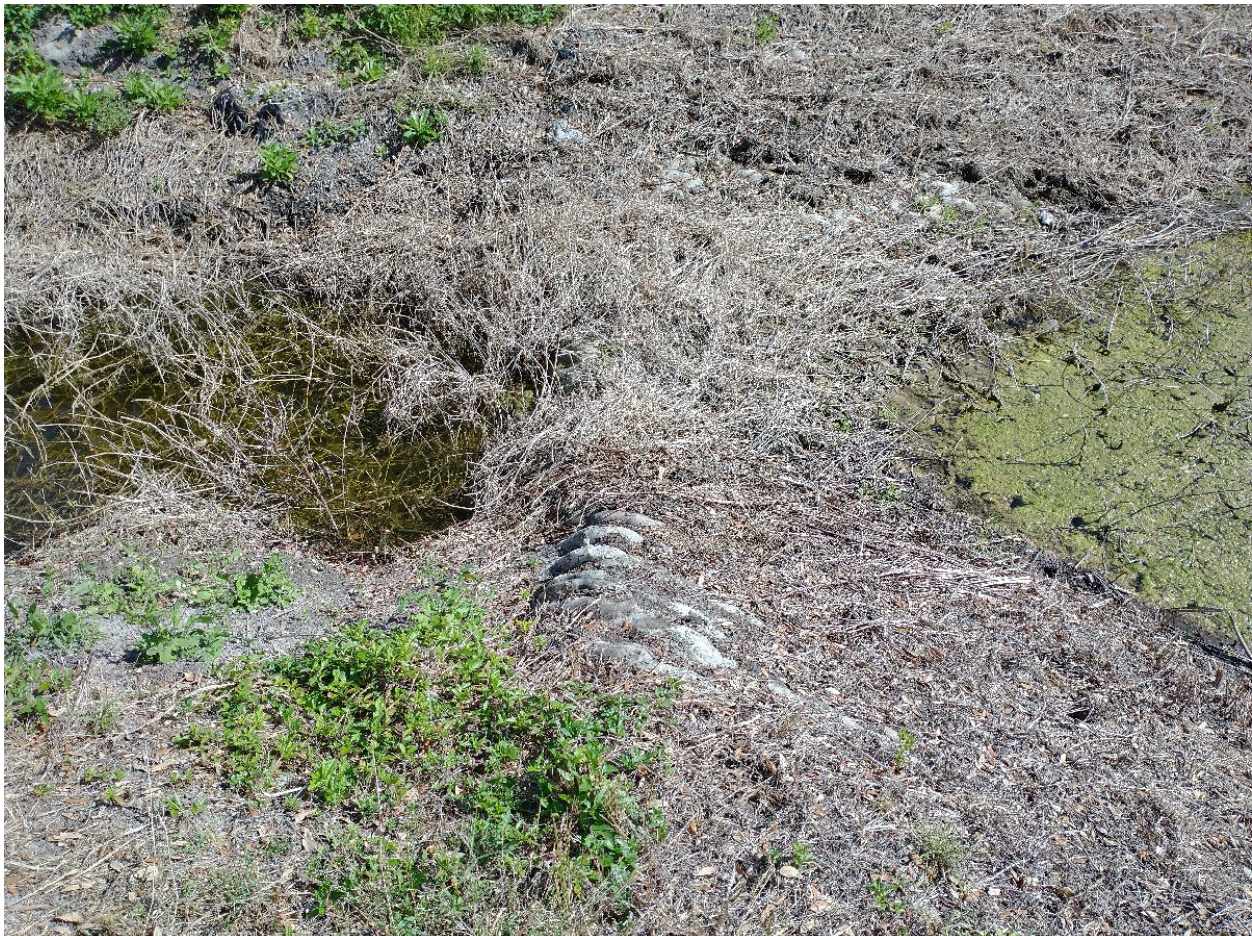
Photograph 11. A concrete erosion-control apron (photograph 11) from 28^{\circ} 33' 5.1'' N 81^{\circ} 37' 14.2'' W, looking southeast from the northern side of the ditch across the apron on March 3, 2022. The apron functions as a weir, controlling the flow of water from the Johns Lake watershed, toward a former water control structure (photograph 9) to a ditch that drains to Lake Apopka (photograph 8).
