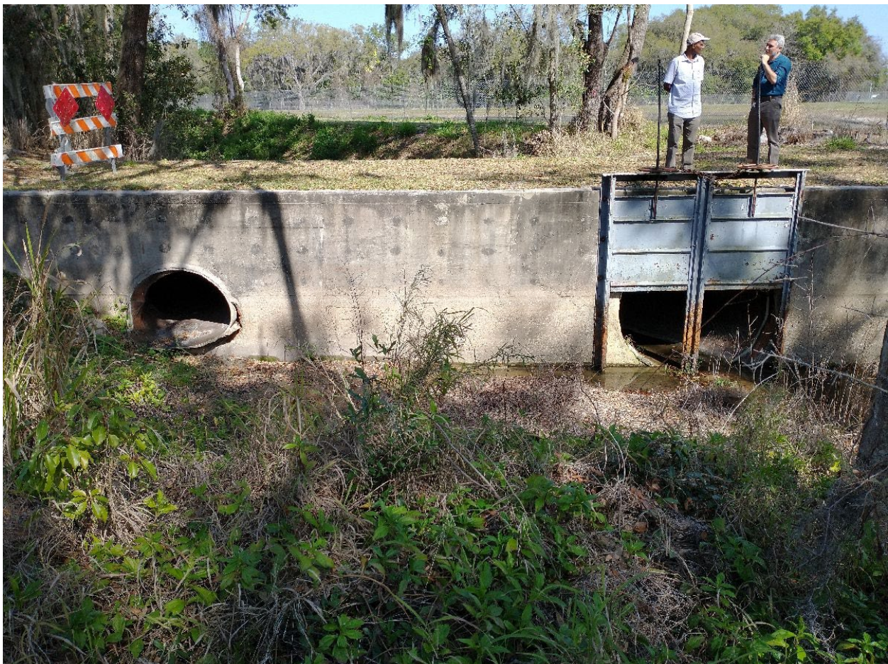
Photograph 9. The upstream side of a water control structure (photograph 7) from 28^{\circ} 33' 5.3'' N 81^{\circ} 37' 14.3'' W, looking northeast, away from West Colonial Drive and toward Lake Apopka on March 3, 2022. The water control structure once regulated the flow of water from the Johns Lake watershed to a ditch that drains to Lake Apopka.
