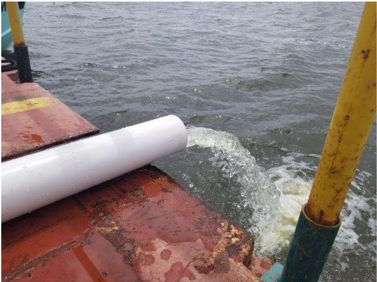
Discharge of clarified water to Lake Jesup.
