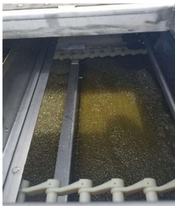
Flotation chamber showing float blanket skim bar.
