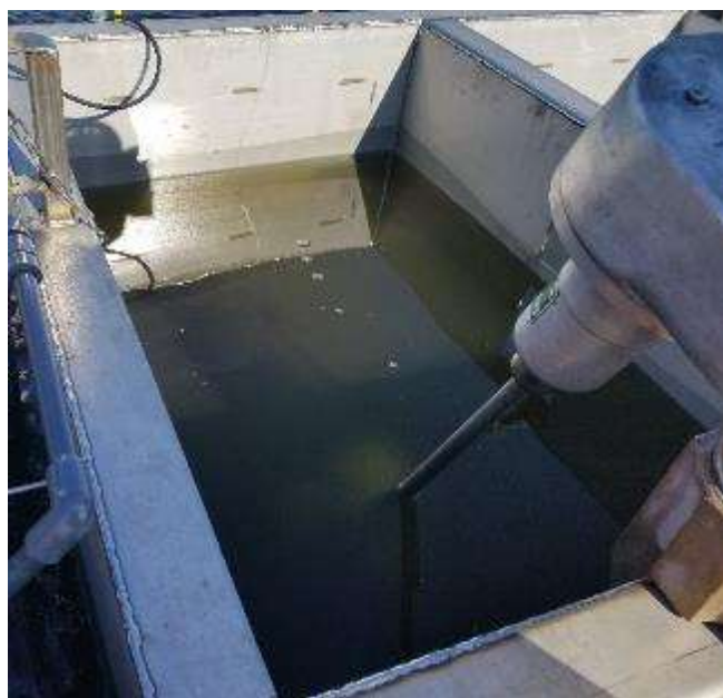
Coagulant chamber showing mixer.
