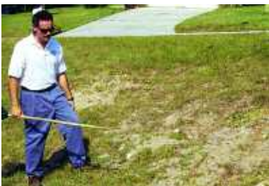
Repair eroded slopes.
