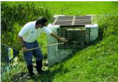
Clear or clean inflow/outflow structures.
