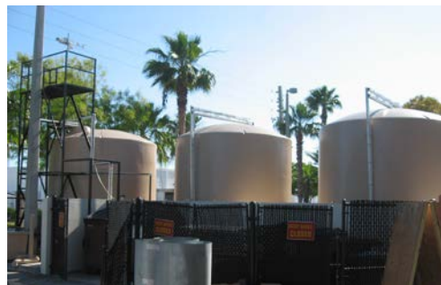
Storage containers for harvested rainwater
