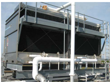
Figure 8. A large capacity cooling tower.
