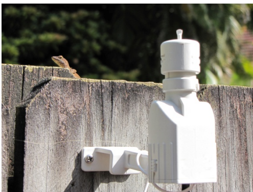
Figure 20. A standard rain sensor.
