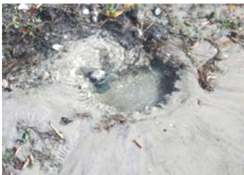
Figure 16. Broken piping underground causing puddling and erosion.
