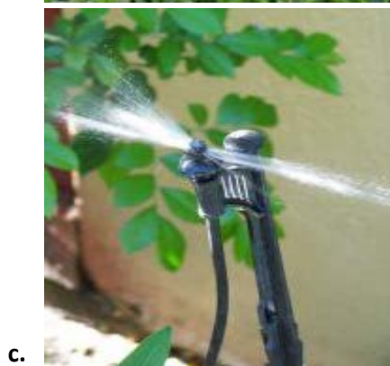
Figure 12. The three main categories of irrigation sprinklers: a) rotor, b) sprayhead emitter, and c and d) micro-irrigation emitters.
