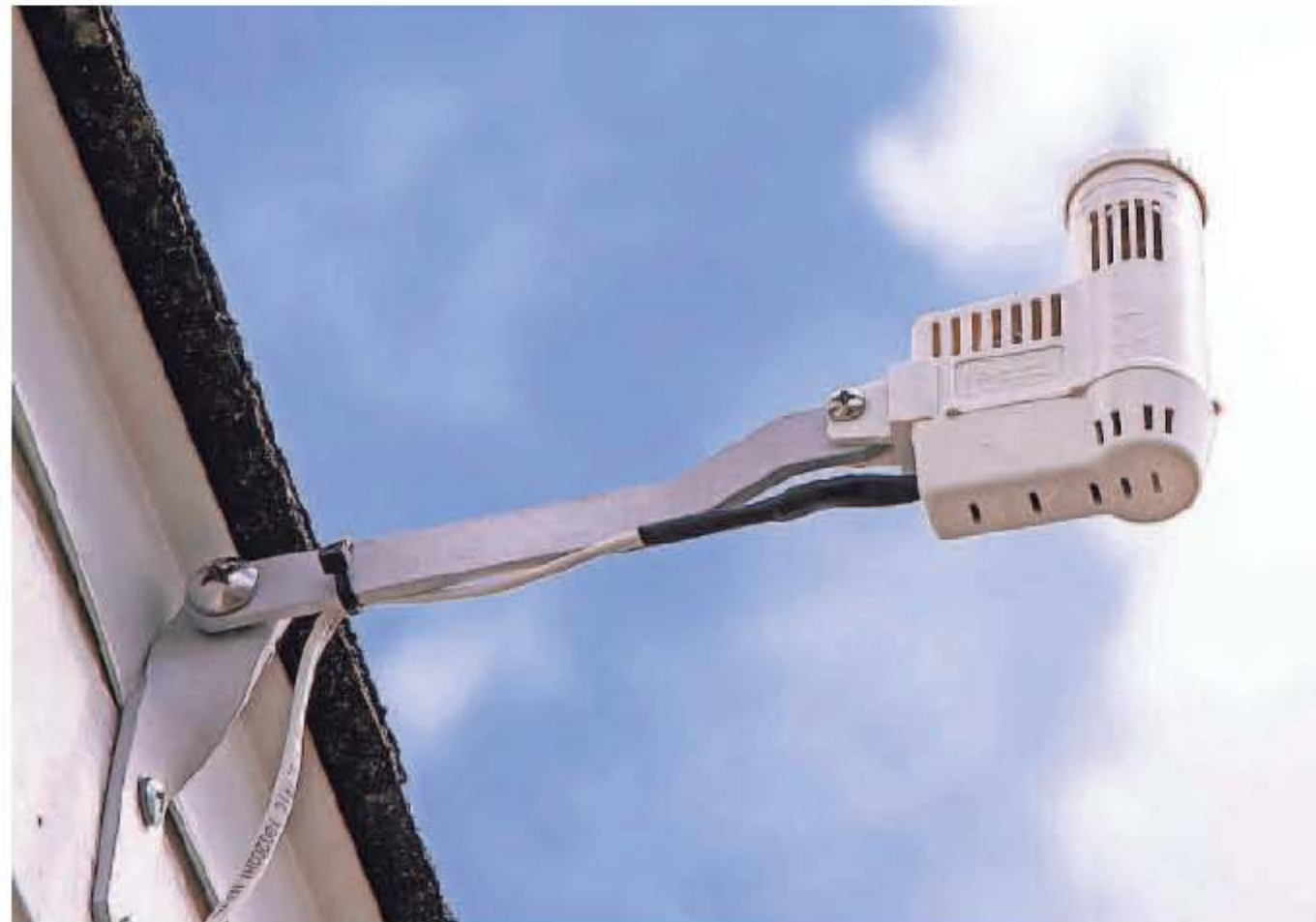
An irrigation rain gauge is mounted to the fascia of a home in Weybourne Landing on Tuesday. On Top of the World, Stone Creek and Calesa Township are implementing many water conservation measures in new homes.
