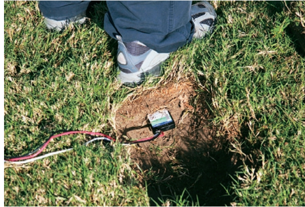
Figure 18. Compaction of soil around sensor to reduce void space and ensure adequate connection between SMS probe and soil
