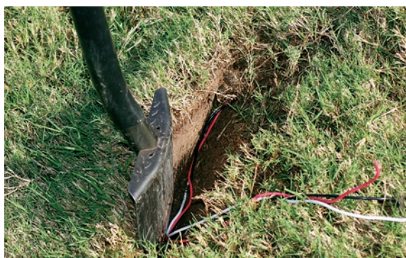
Figure 26. Placing sensor wires while continuing to lift the trench
