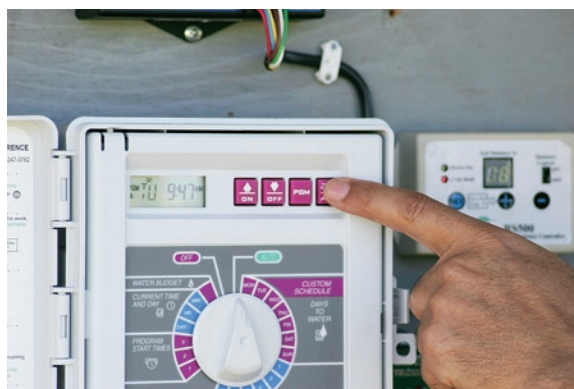
Figure 41. Manual start of irrigation timer while SMS controller is “on hold” to test proper operation
