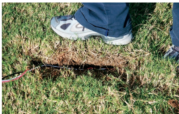
Figure 25. Closing the lift trench
