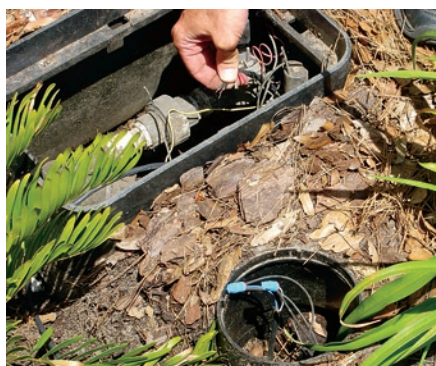
Figure 32. Prepare the soil moisture sensor and zone valve for connection
