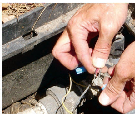
Figure 33. Connect the wires from the soil moisture sensor to the zone valve
