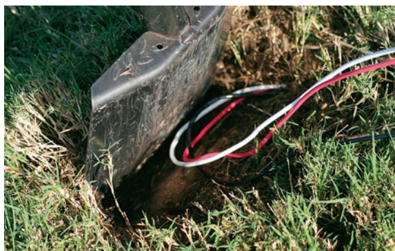
Figure 24. Lifting shovel within the lift trench to create room for SMS wiring
