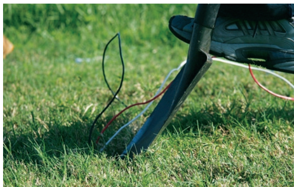
Figure 23. Beginning lift trench
