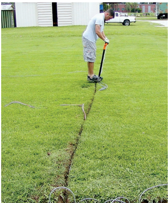
Figure 27. A conventional slit trench should only be used when placing wiring in conduit
