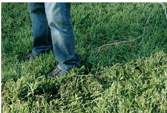
Figure 14. Gently compacting the turf grass area
