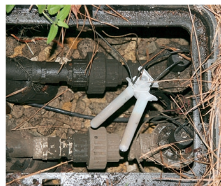
Figure 34. Enclose all wire nuts in direct burial connectors
