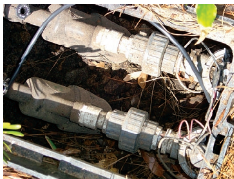
Figure 30. Uncover the irrigation zone valve box
