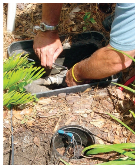
Figure 31. Disconnect the existing wiring connection between the irrigation timer and zone valve
