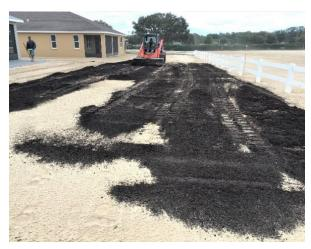
Figure 1. Spread compost with front-end loader. Credit: UF/PREC.
