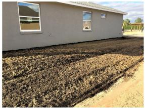
Figure 3. Check for a general 6-inch incorporation depth, 4-inch minimum in small areas and level the amended surface after compost incorporation. Credit: UF/PREC.
