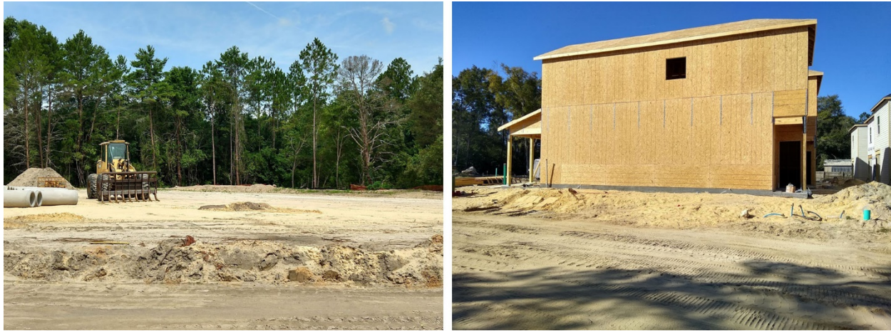
Figure 4. Clear cut residential site after removal of topsoil; imported sand fill under house foundation slab. Credit: UF/PREC.
