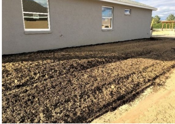
Figure 13. Level the amended surface after compost incorporation. Credit: UF/PREC.
