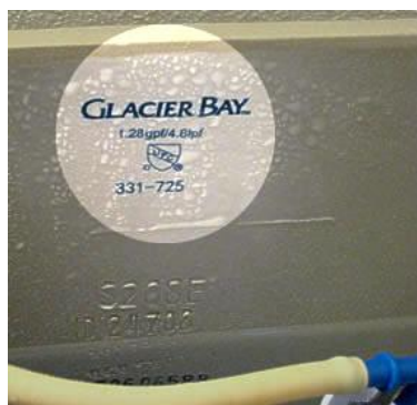
A stamp with the performance values located inside the toilet tank.
