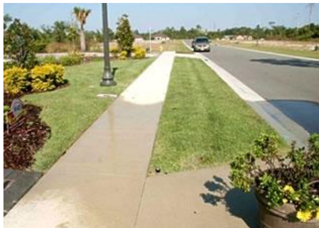
Unacceptable overspray is to be minimized
