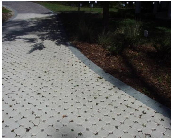
Permeable surface driveways (Photos courtesy of UF IFAS)
