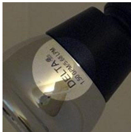
The flow rate stamp is clearly visible on this showerhead
