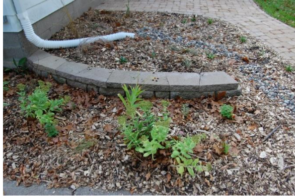
Downspout extender (Photos courtesy of UF IFAS)
