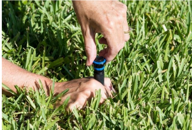
Installing a new spray nozzle
