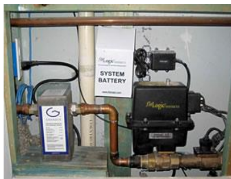
This whole-house leak detection system is an example of indoor innovation
