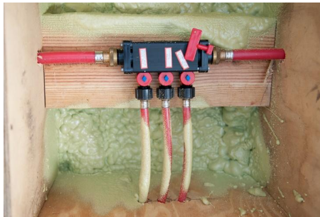
Manifold plumbing system
