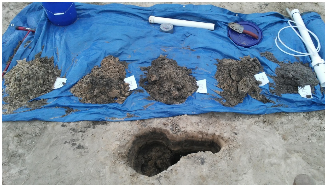
Figure 2-10. Excavated soil cavity (lower center) for installation of lysimeter (upper right). Lifts were separated and ordered (1-5) to reconstruct soil profile after installation.
